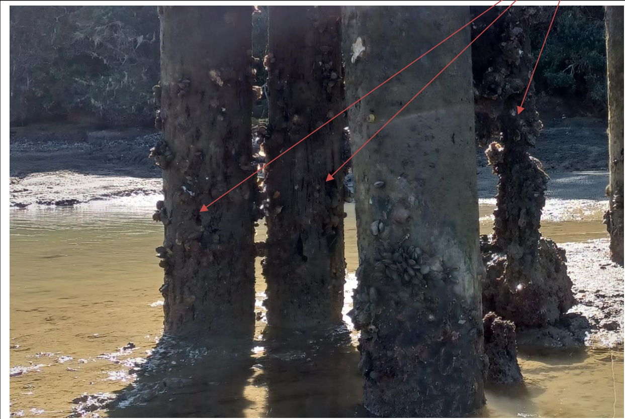
Pile displaying severe worm / Bore damage
