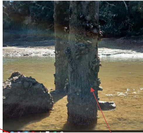
Pile displaying severe worm / Bore damage
