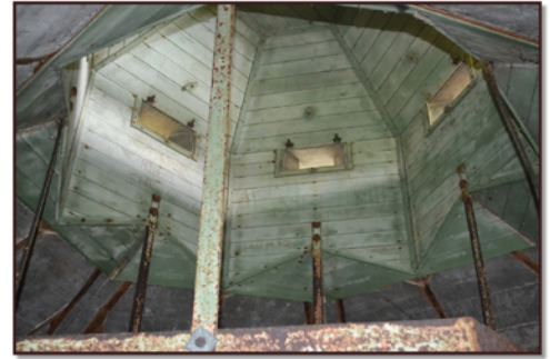
Whangaroa mine observation post Source: Heritage New Zealand, Pouhere Taonga
